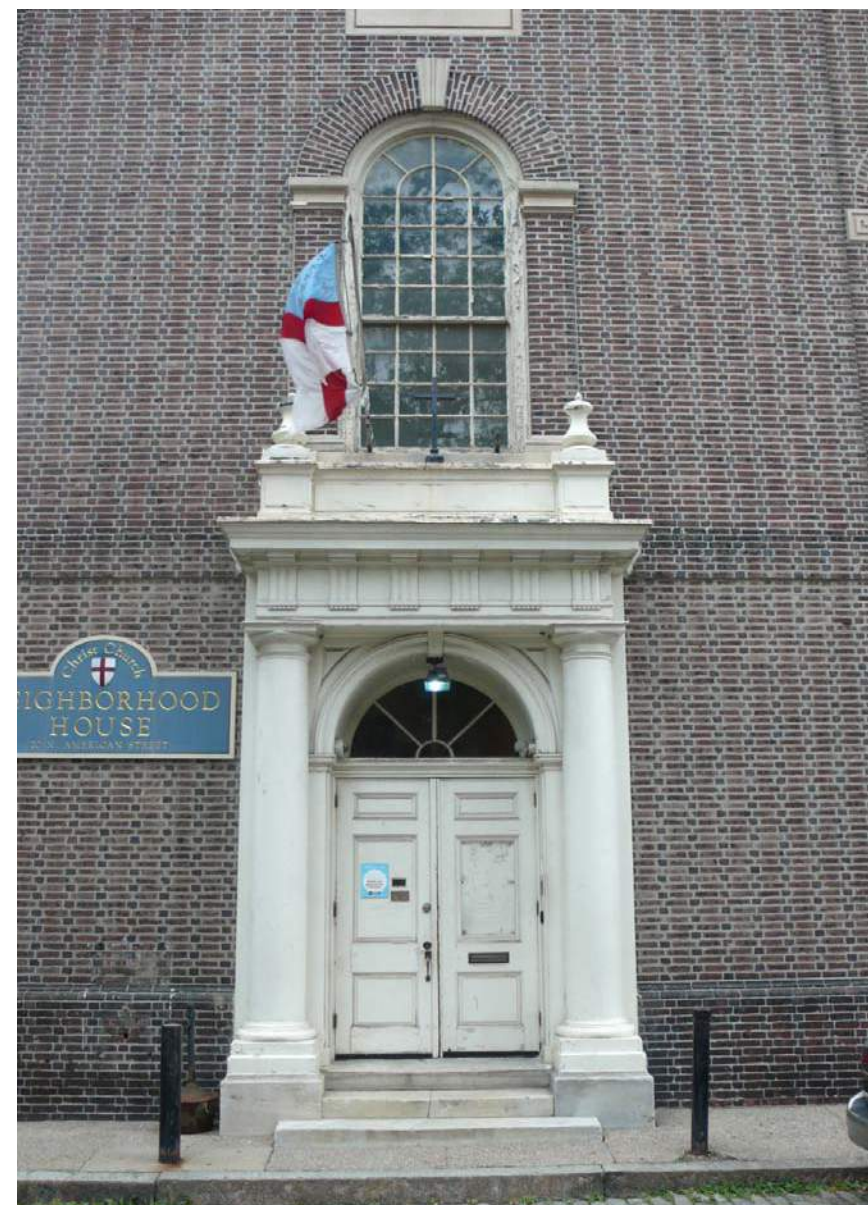
Large scale entries at civic and cultural buildings
